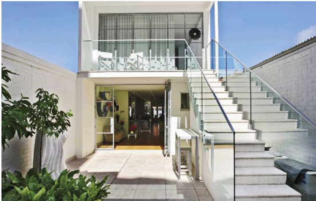
The mod courtyard of Costa Plenti, a private apartment for those seeking villa comforts, Sydney-style
